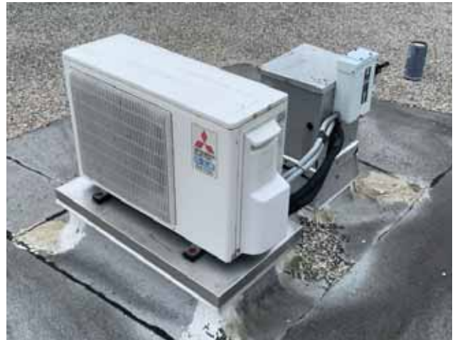
22 - DUCTLESS SPLIT SYSTEM COMPONENT
